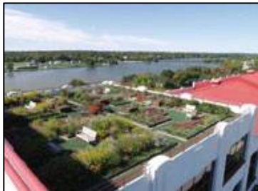
Green Roof, Weston, Inc.
