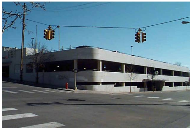
1 st & Washington, pre-demolition (looking south-east)
