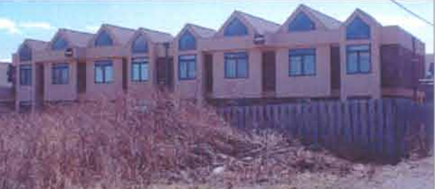
CONIFEROUS TREES, AS WELL AS SINGLE AND MULTI STORY OFFICE AND MEDICAL BUILDINGS, BORDER THE SOUTH END OF THE SITE.
