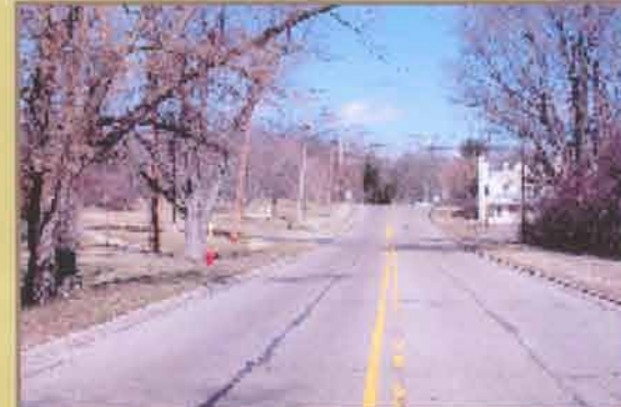
VIEW FACING SOUTH ON PLATT, A TWO-LANE, 25 MPH ROAD THAT BORDERS THE WEST SIDE.
