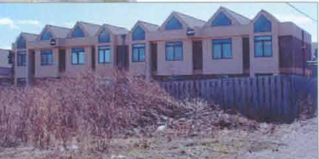
CONIFEROUS TREES, AS WELL AS SINGLE AND MULTI STORY OFFICE AND MEDICAL BUILDINGS, BORDER THE SOUTH END OF THE SITE.
