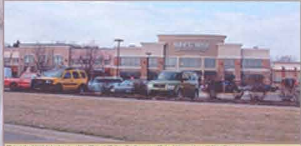
EXISTING DEVELOPMENT ACROSS WASHTENAW IS SUBURBAN IN CHARACTER WITH LARGE SETBACKS AND EXPANSIVE PARKING LOTS.
